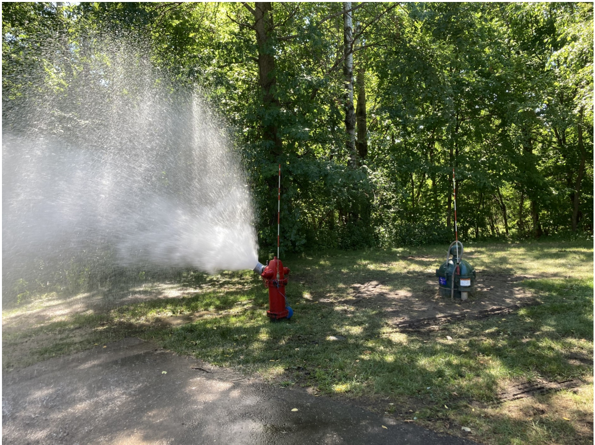
Flushing of the chlorinated water used to disinfect the well prior to putting it back into service
