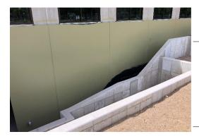
Waterproofing behind the stonework is installed at the exterior stairs.
